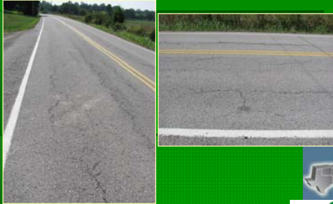
Hickman Co. Existing Surface
