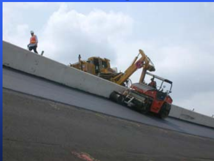
Compaction Against Wall
