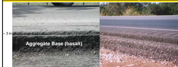
Thin-surfaced, "flexible" pavement
